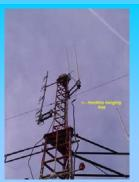
After repairs were made high intermittent VSWR was noted so the output was switched to a tri-band back up antenna and the problem seems to be cured.
